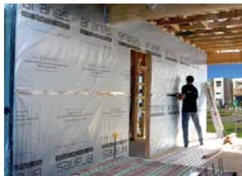
Ametalin SILVERBRANE Reflective High Permeance Wall Wrap Photo: Ametalin
