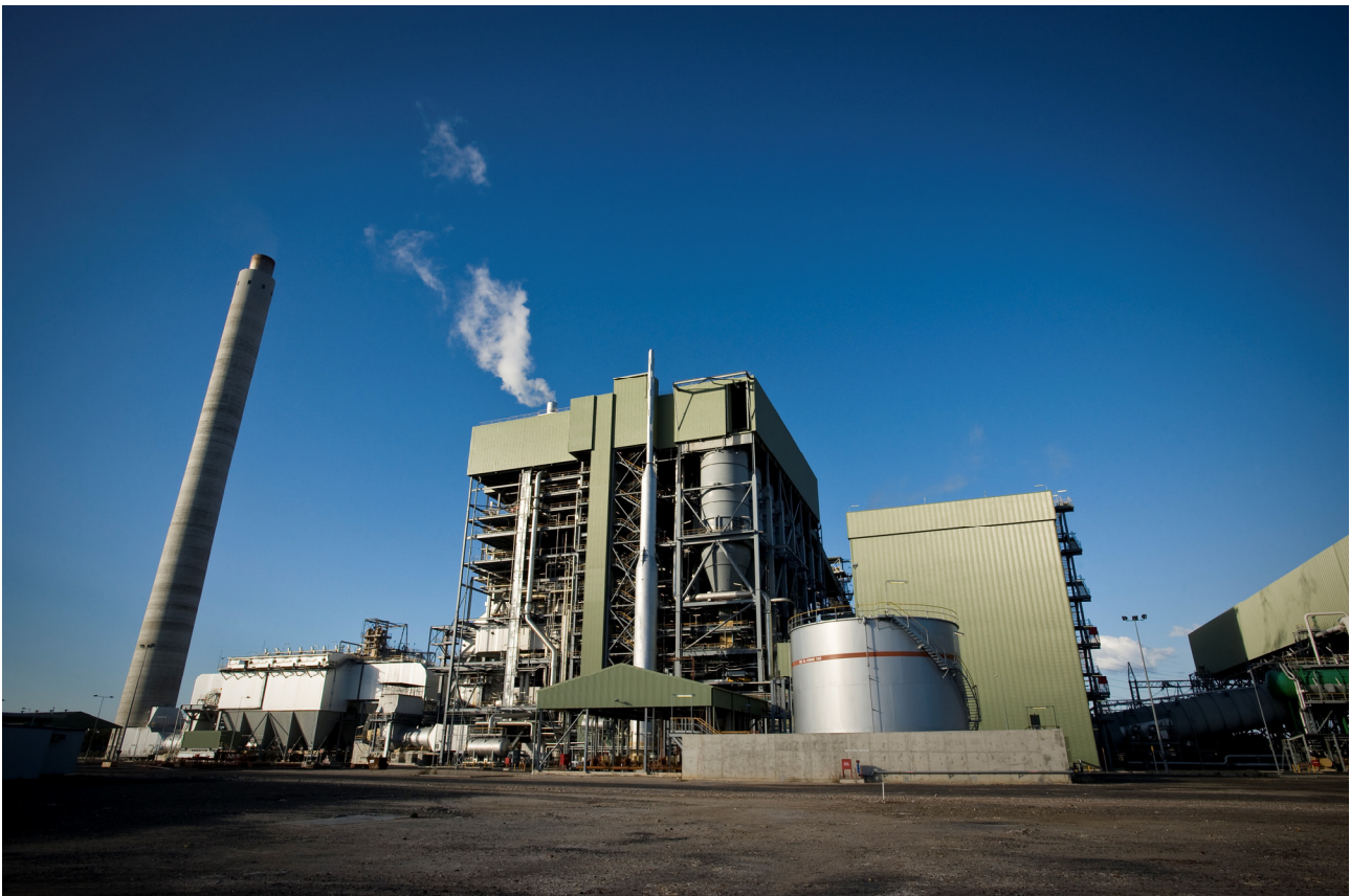
> Kogan Creek Power Station.
